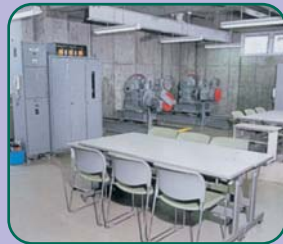
Elevator Machine Room
